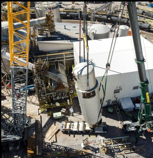
Mountain recently performed a turnaround project that involved our LR1600 crawler and LTM1750 all terrain cranes. The highlight of the event was removing a cold reheat exchanger and replacing it with a new one. We even got our SMPT Goldhofer trailer in the mix!
