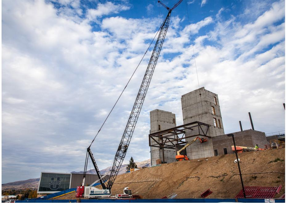
Mountain Crane is thrilled at the opportunity to help with the construction of the new Maverik Stadium at Utah State University in Logan, Utah. Mountain Crane is currently providing the crane for the erection of the steel for the press box structure using our Linkbelt 278 300t lattice truck crane.
