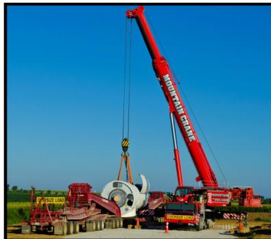
The last job featured was for Wanzek Construction in Adair, Iowa. Several nacelles weighing 195,000 lbs. each had to be unloaded from trucks and then set carefully onto the ground.
