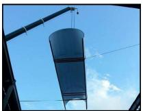
This lift required intense precision as there was about a 1-inch clearance on both sides as they lifted the tunnel from the ground and into its proper position through the open ceiling into the aquarium. Our talented crane operator, Riley Allen, executed this lift flawlessly. Check out the following video clip from KUTV for more information about this project.
