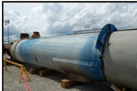
The heaviest of the lifts was 551,000 lbs., which was walked into the unit and set at a 85 ft. radius. The second heaviest lift was 530,000 lbs. set in place at a 95 ft. radius.
