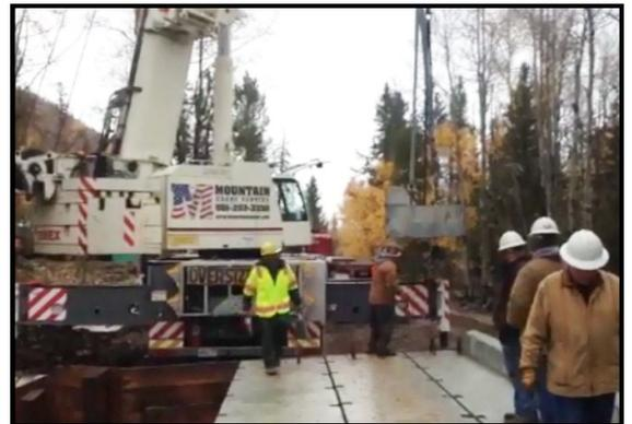
A similar project was needed at "Hole in the Mountain Trail" out of Lonetree, Wyoming. In order to place the crane into its positions for capacity lift, trees were tied back for the counter weights and rear swing to be possible. It took a lot of extra planning and coordination to not damage these beautiful environments, but Mountain Crane executed the project effectively with no delays.
