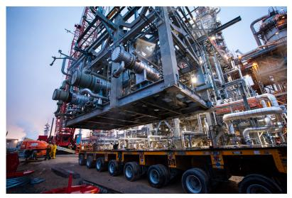
towoc 2250 with MAXER-2000. Mountain Crane's team designed over 21,000 pounds of rigging to allow for quick transitions between the different modules and varying numbers of picking points. After lifting the modules off of the Goldhofer trailers, the Manitowoc 2250 pivoted and tracked into the crude unit while suspending the modules over existing refinery structures. Due to expert planning
