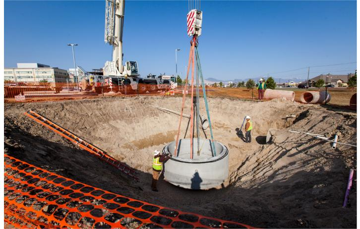
Earlier this month, Mountain Crane Service worked with Reynolds Parson to install box culverts at Riverton Hospital. Using our Demag 170t and a Grove RT 90t, we were able to successfully set the 38,000 pound culverts.
