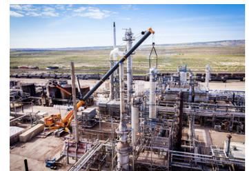
In August, Mountain Crane utilized the new Liebherr 1750t crane to place the new [LEF tower](#) in Sinclair, Wyoming.
