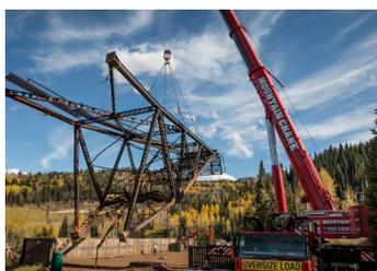
Mountain Crane moved a [broken mine tressil](#) back to its original location. The tressil is 85 feet tall and weighs 76,000 pounds.
