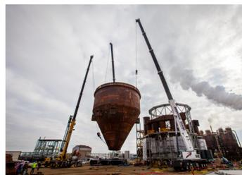
Mountain Crane performed a [unique lift](#), using a Grove 550, a Liebherr 500, and a Grove 275 to place a spray dryer filtration system.
