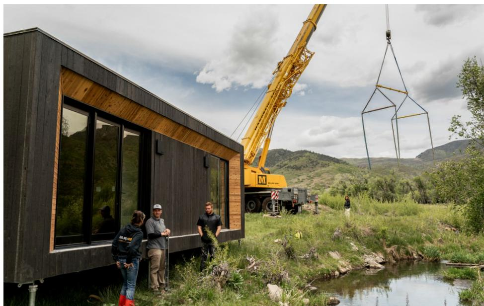
Talk about a quick turn around! This home was built completely in a factory, brought to the site, and our team did the heavy lifting. Our 200 ton crane and crew installed this modular home in no time at all, leaving the structure move-in ready! The home was built by Modal Living and is totally customizable for cabins, rentals, and recreation. Glad to be a part of this scenic job site!
