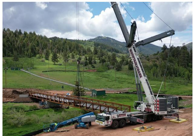
Our team soaked in the gorgeous views of Park City recently as our 500 ton crane hoisted two bridge sections into place. The first weighing in at 35,000 lbs and the second at 55,000 lbs.
