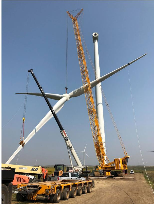
Mountain's crew was on-site to handle the rotor and main bearing for a wind turbine tower near New Salem, ND.
