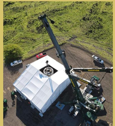
Generator was carefully rebuild within the enclosed tent.
