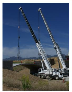
Mountain Crane Service recently set a pedestrian bridge in Daybreak for Ralph L Wadsworth Construction. The Oquirrh Creek Bridge was set in two pieces, each section weighing 38,000 lbs.
