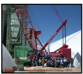
14000 220 ton crawler crane and Manitowoc 777T 220 ton conventional truck crane were utilized on this project.
